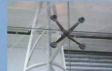
• Fixed Support 12mm Clear Tempered Glass
